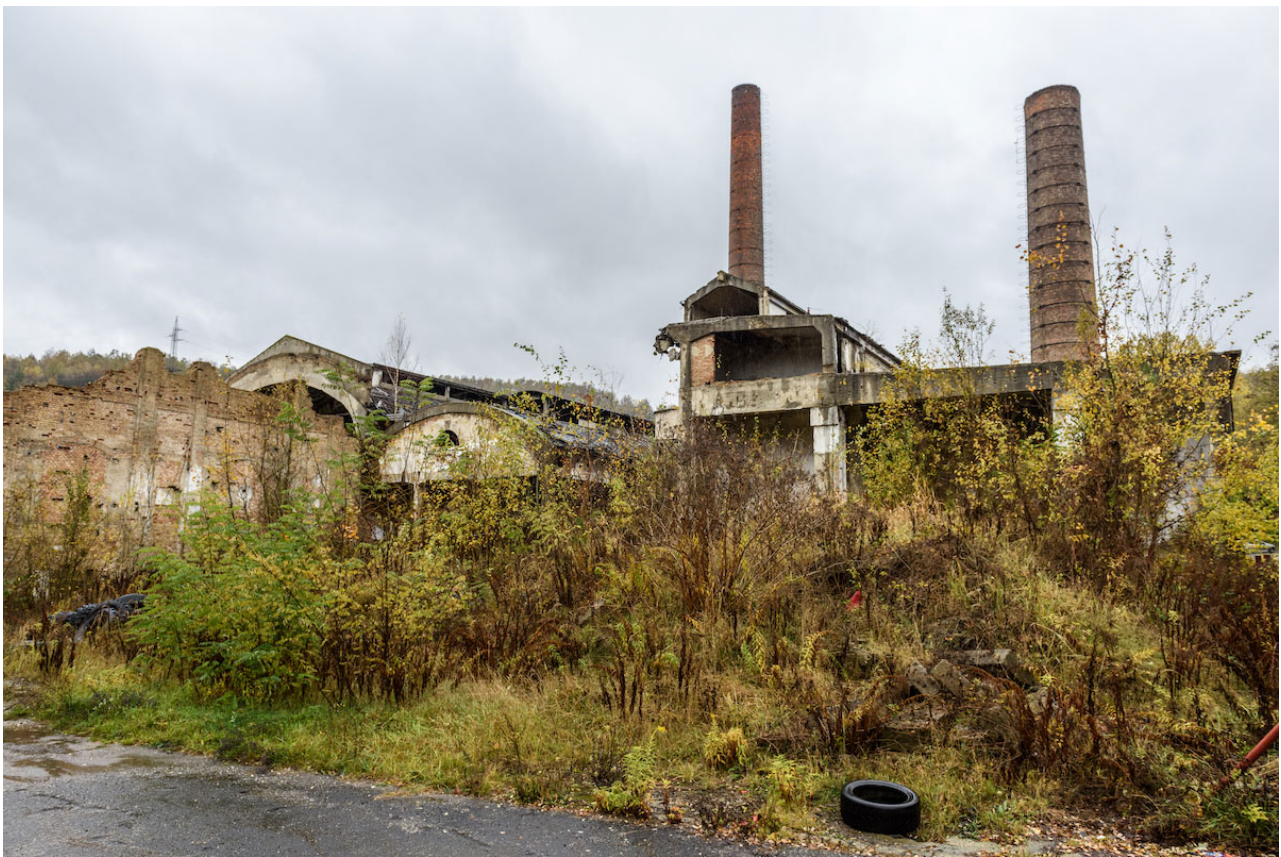
Figure 5: Reka Komoli: Former Soviet power station, 2018
