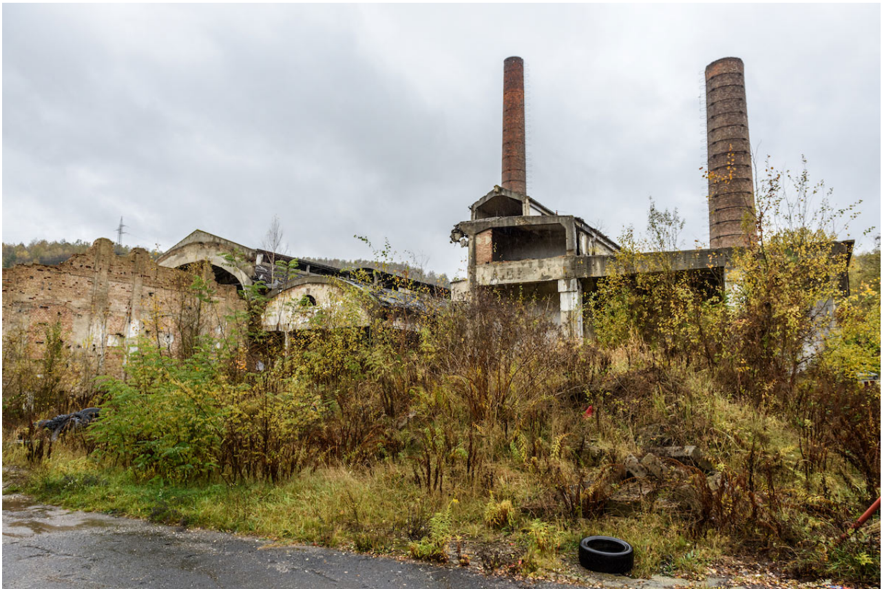
Figure 5: Reka Komoli: Former Soviet power station, 2018
